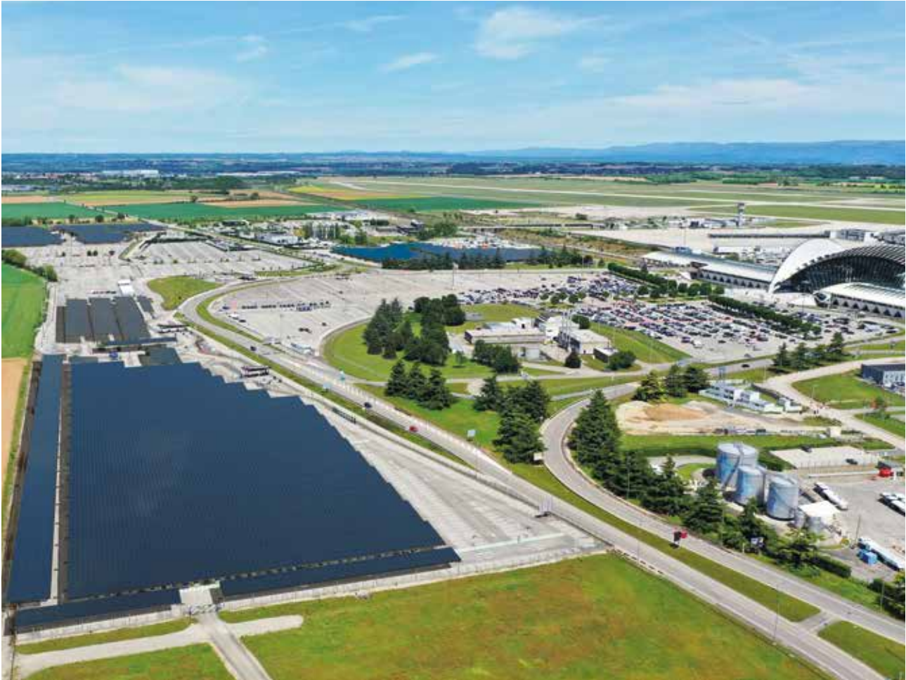
At Lyon-Saint Exupéry airport, the VINCI Concessions subsidiary SunMind partnered with Neoen to deploy one of France's largest solar canopies, spanning 14 hectares, with a capacity of 20 MWp (computer-generated image).
