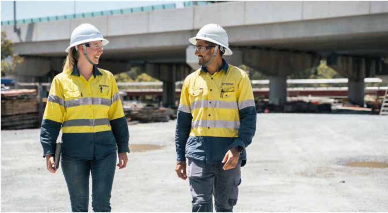
Seymour Whyte is leading the project to upgrade the M1 Pacific Motorway between Palm Beach and Tugun in Australia.
