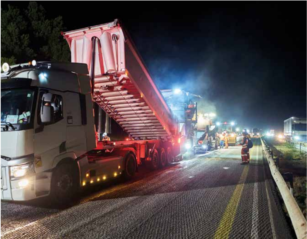
On the A61 resurfacing project between Carcassonne and Lézignan, a significant portion of the asphalt pavement from the old road was reused in the new one.
