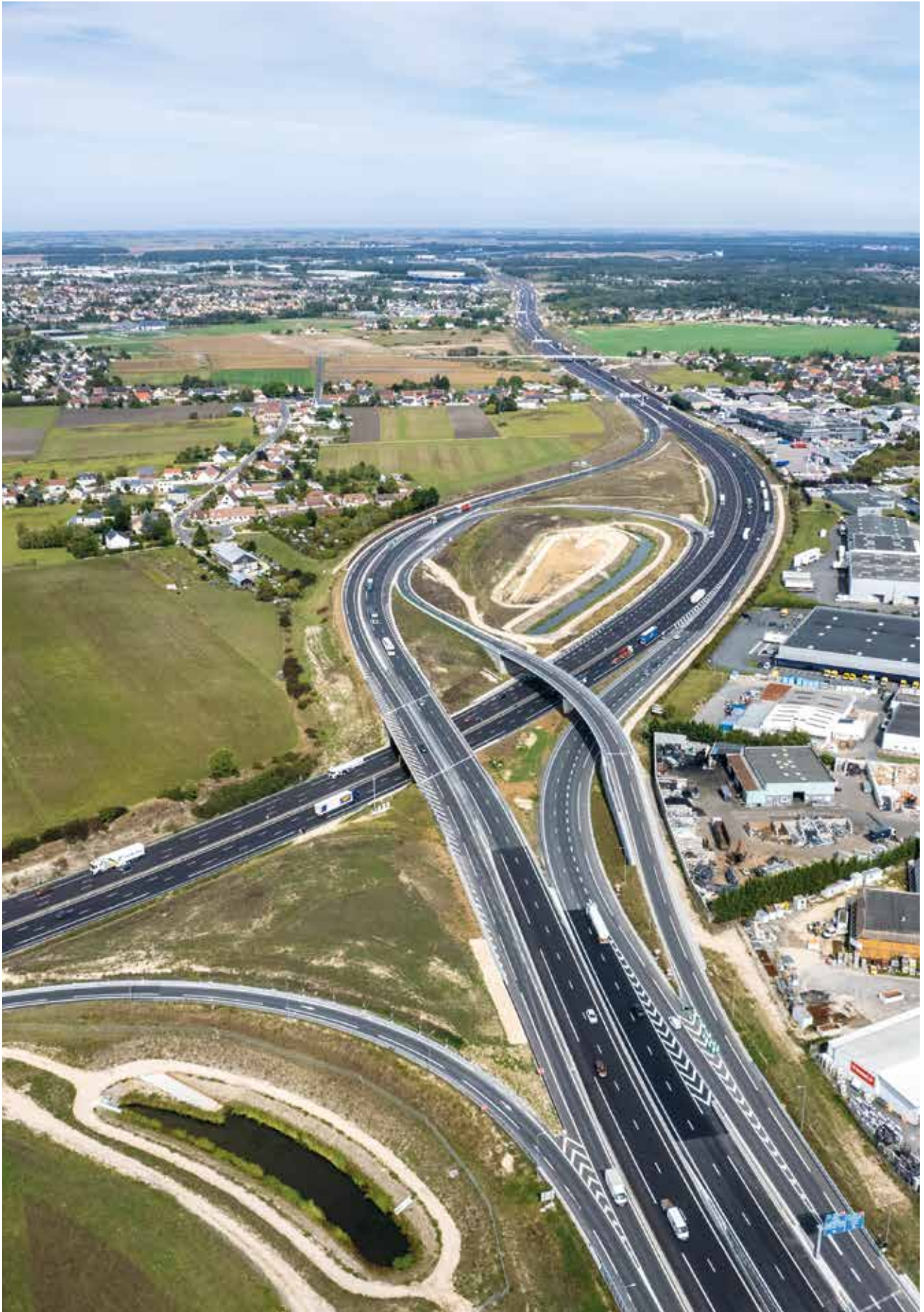
Redesign of the A10/A71 junction north of Orléans, completed as part of the motorway stimulus plan. This project included creating a fourth lane on the A10 in both directions of traffic.
