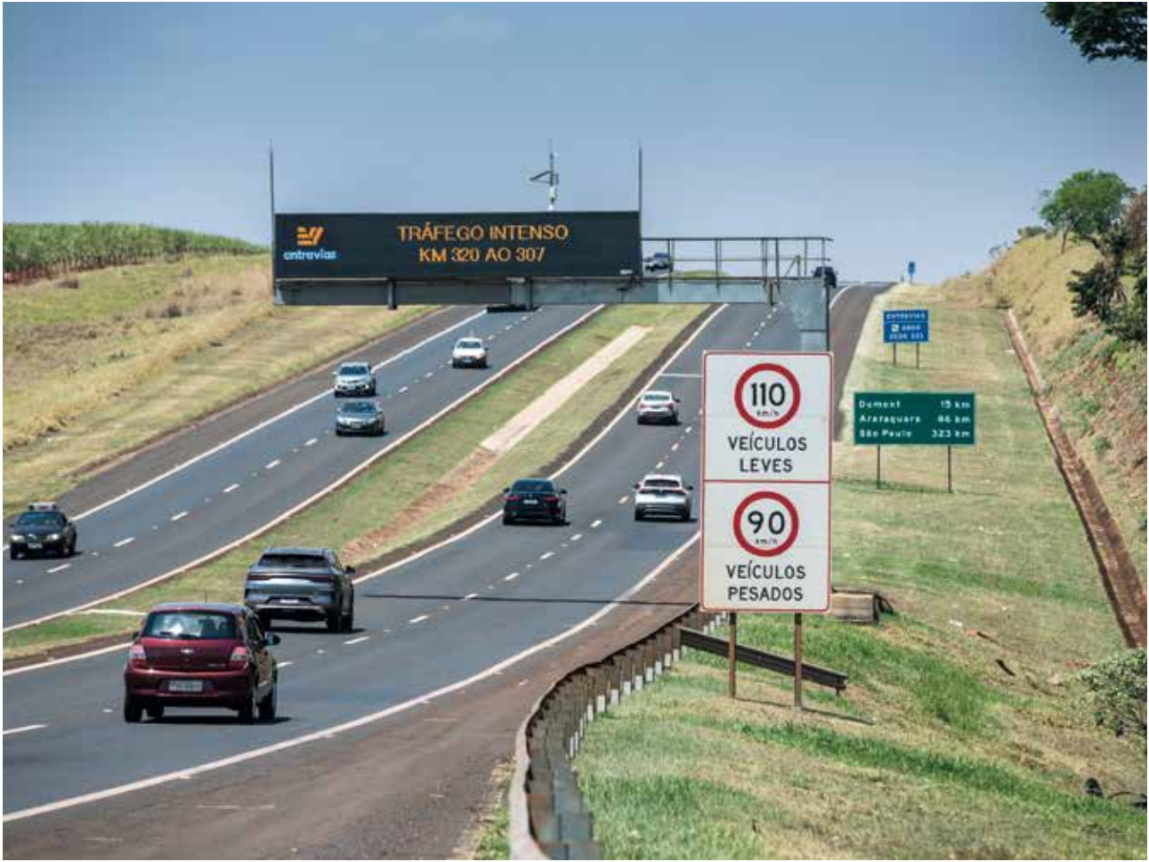
With the acquisition of 55% of Entrevias in Brazil, VINCI Highways, which already holds the concession for the Bogotá–Girardot highway in Colombia and the Lima ring road in Peru, continues to develop in South America.
