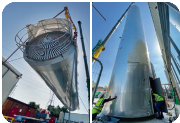
Thermal store installation taking place at our Beckton site, part of the new heat recovery system to improve energy efficiency and cut carbon emissions.
