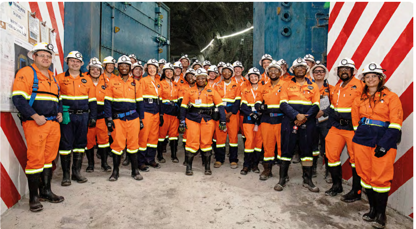
Below surface: the Sustainability Committee and senior leaders met with site management and employees underground to see the progress being made as Venetia transitions from being a surface mining operation to an underground mine.
