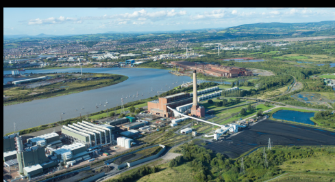
Uskmouth power station
