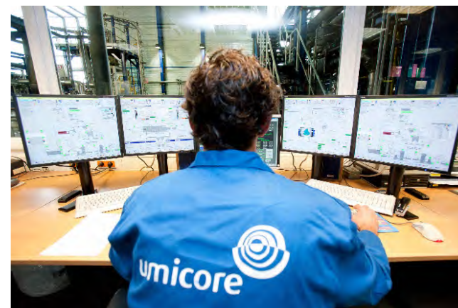
Umicore Precious Metals Refining leaching and electrowinning in Hoboken, Belgium
