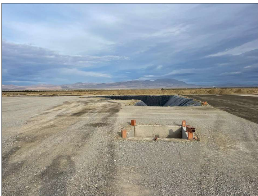
MOU-2 well pad construction
