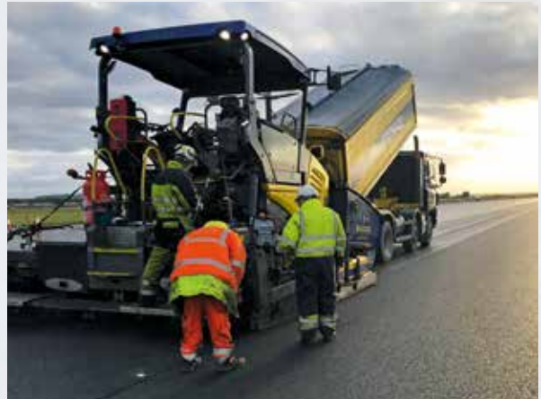
Above: Runway resurfacing at RAF Kinloss (courtesy of the Defence Industry Organisation)
