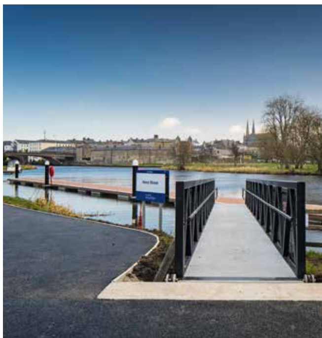
Above: The Henry Street Jetty in Enniskillen, constructed by Whitemountain
