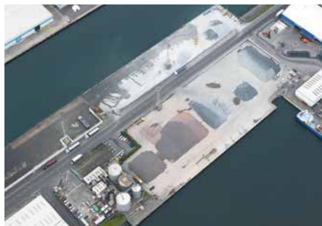
Above: Barnett Dock aggregates terminal, Port of Belfast
