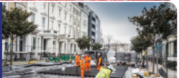
Permavoid installed at Kensington Park Terrace, London
