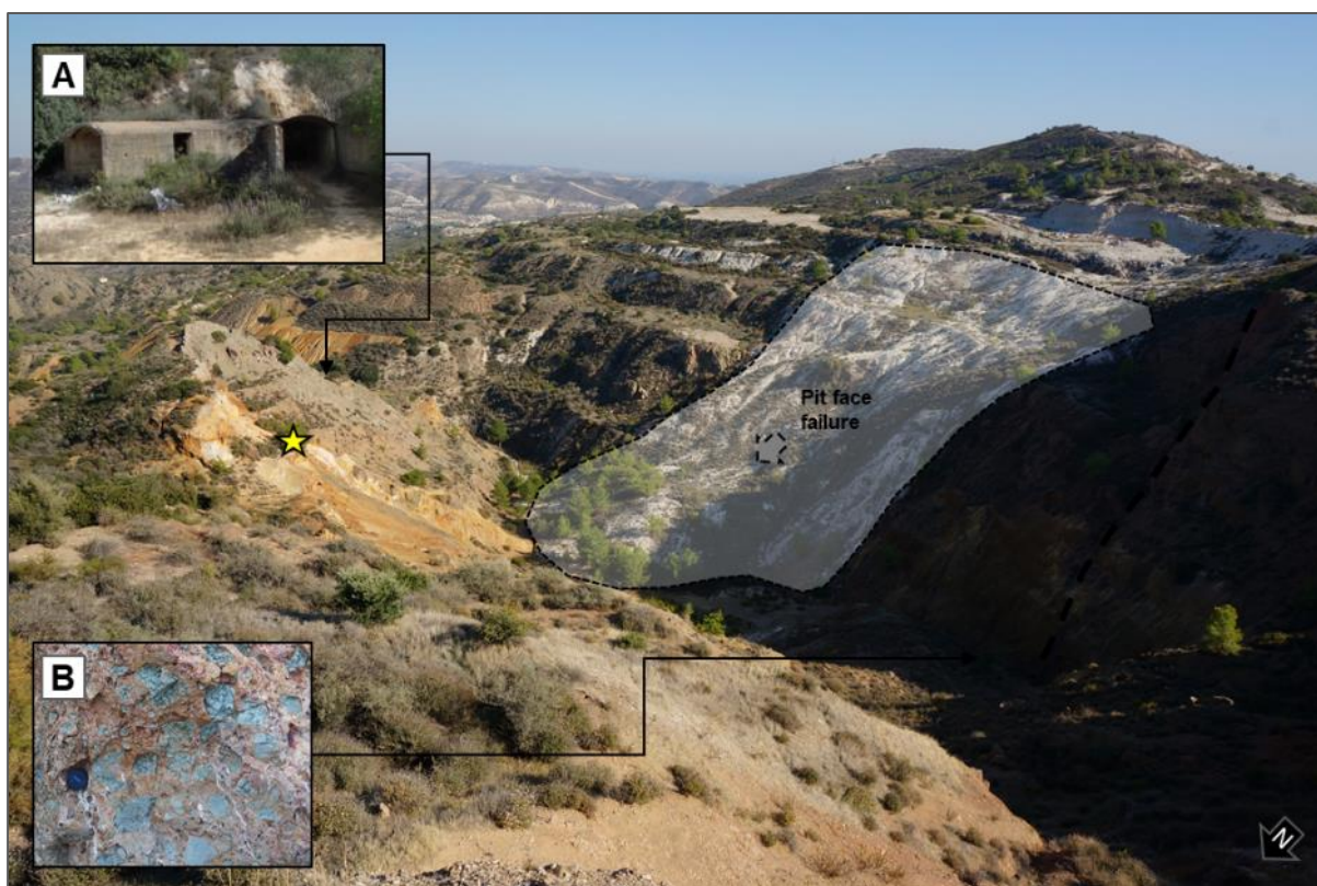
Figure 32 – Mavridhia open pit. Extensive gossans and ochre cap the norther pit wall. Note footwall fault and Lefkara formation landslide. A - Adit entrance to underground workings, assumed to be Kalavassos 'A' at entrance to pit; B - Weathered pillow basalt; Star – cross reference location to Figure 31 (Oct 2018, Andrew Craig).
