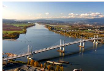
Golden Ears Bridge Canada
