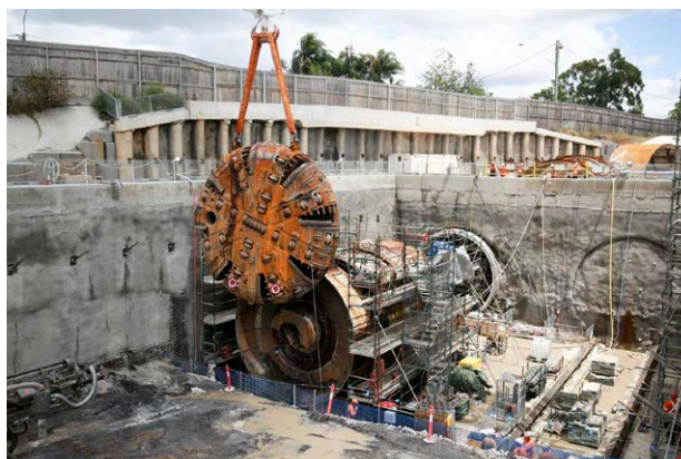
Transport for NSW last tunnel boring machine being retrieved on Sydney Metro.
