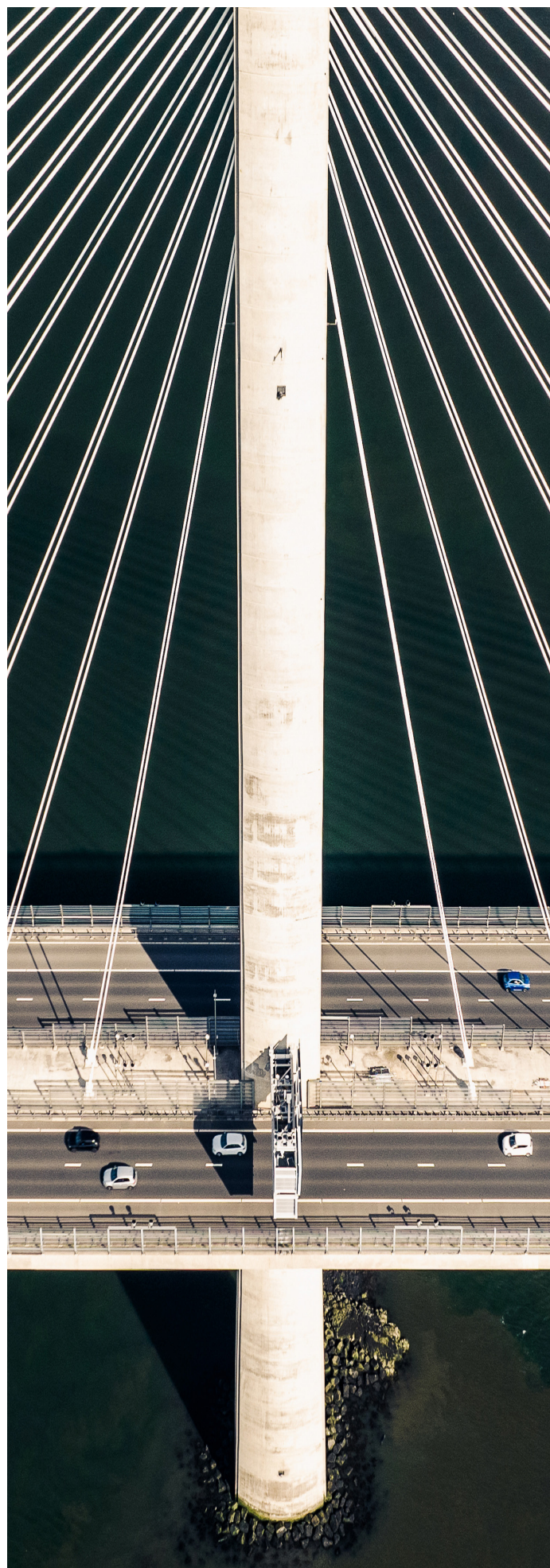
Queensferry Crossing, Scotland.
