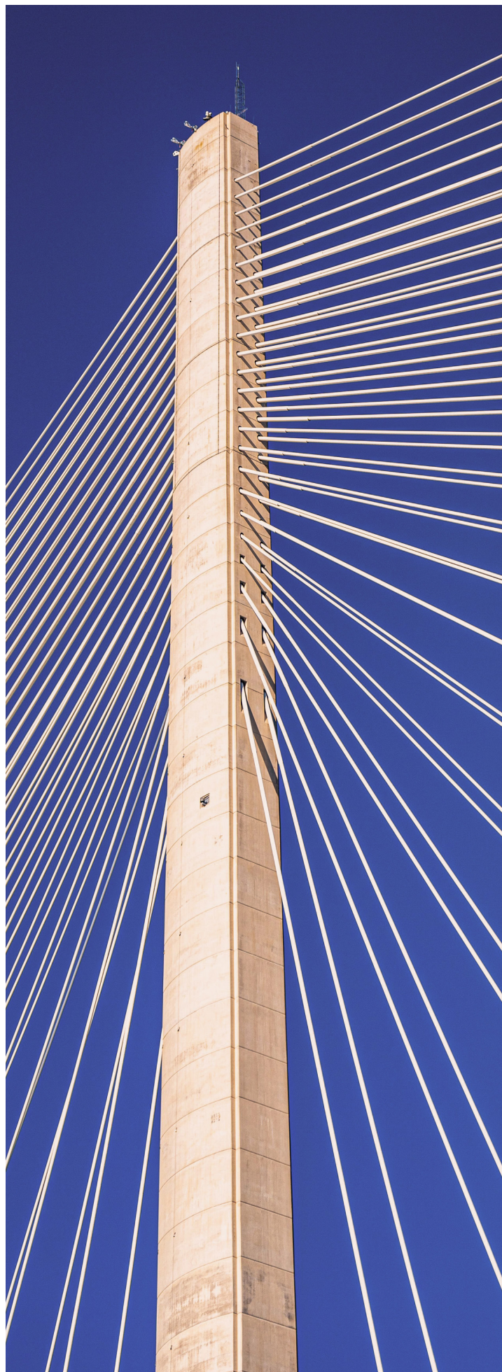
Queensferry Crossing, Scotland.
