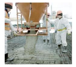
helps to maximise the efficiency of land plot configuration. Compared to construction using prefabricated panels, poured-concrete technology is highly mobile and requires relatively limited maintenance capital expenditure. We are able to do most of the manufacturing on-site instead of maintaining a separate factory for this construction material.
