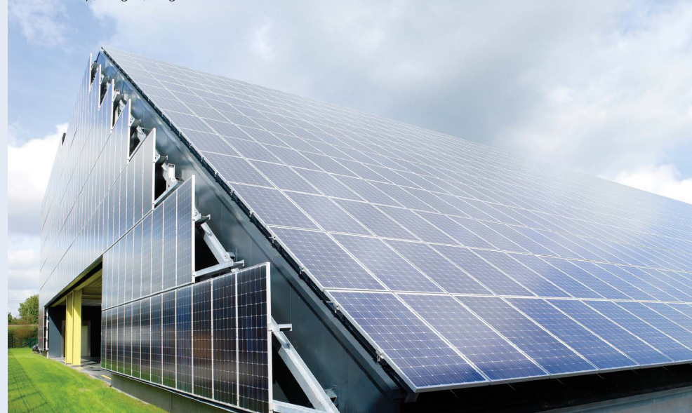
DC Oostkamp, Bruges, Belgium.
