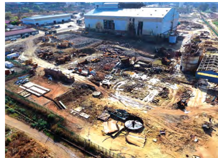
Crown plant demolition activities undertaken to date
