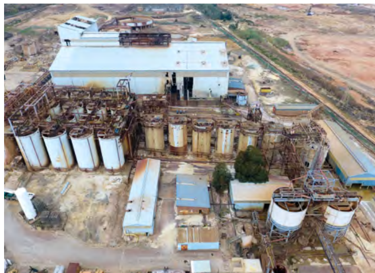
Crown plant prior to demolition
