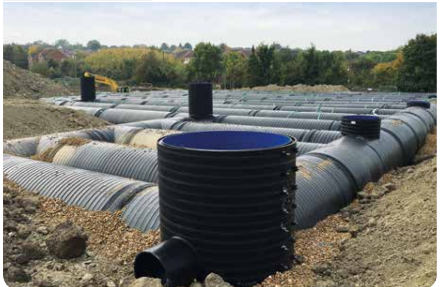
Polypipe's surface water attenuation solution for the Houghton Regis residential development scheme
