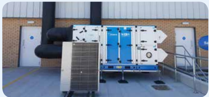
Nuair Boxer Packaged Solutions (BPS) air handling unit
