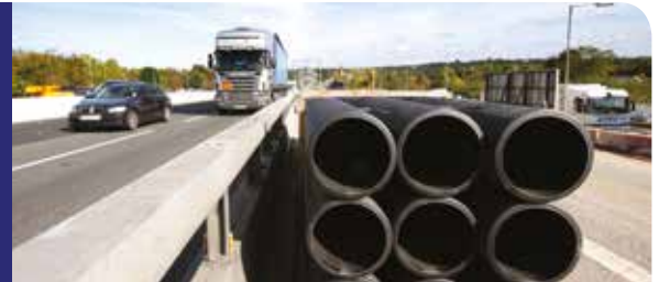
Polypipe drainage solution for M27 road widening scheme
