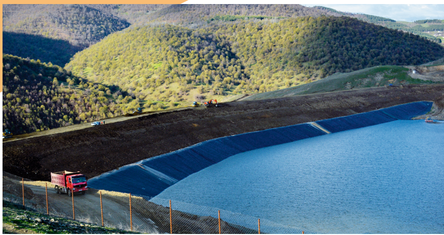
Tailings dam showing the newly raised wall waiting to be lined.
