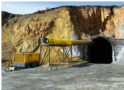
Entrance to the newly developed Gadir decline.
