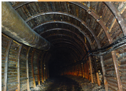
Inside of the Gadir decline showing wall and roof supports.
