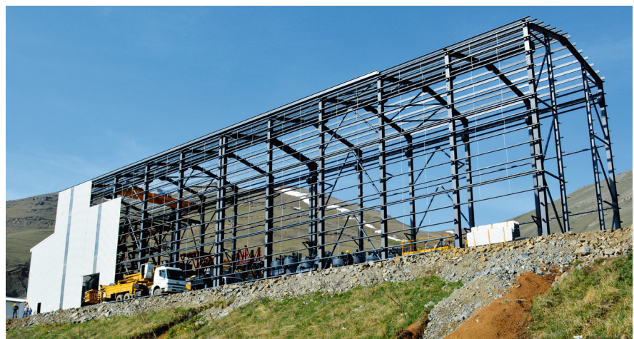
The new small scale flotation plant which is under construction.
