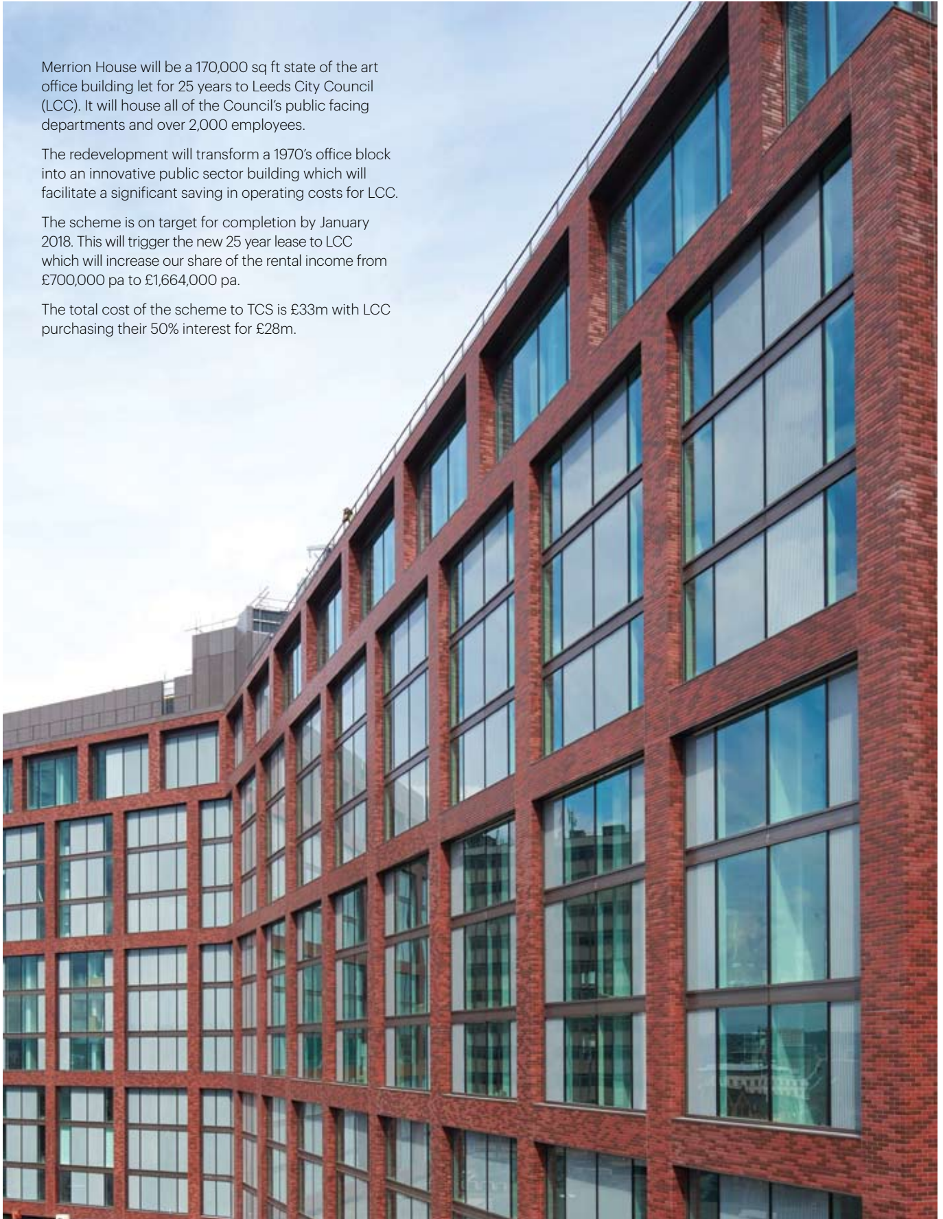
Refurbished Merrion House
