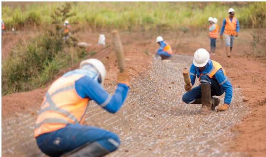
Erosion control measures at Rio Doce floodplains.
