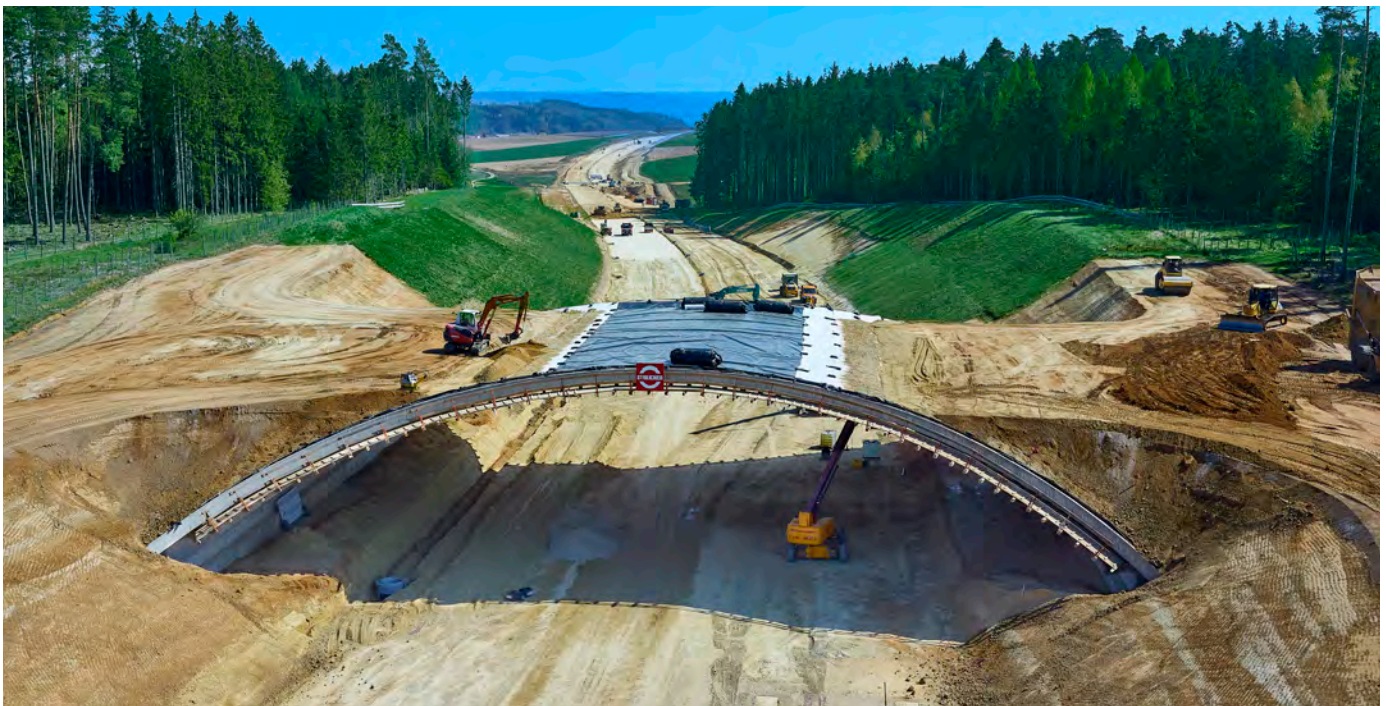
OPTERRA, part of CRH's Europe Materials Division, supplied concrete for this 'green bridge' on the Bundesstraße motorway project in Southern Bavaria, Germany. The project, which runs through a forest area, includes a new motorway as well as 14 additional structures. The green bridge, completed in May 2019, will enable wildlife to cross the busy motorway, thus reducing the impact of the project on the area's biodiversity.
