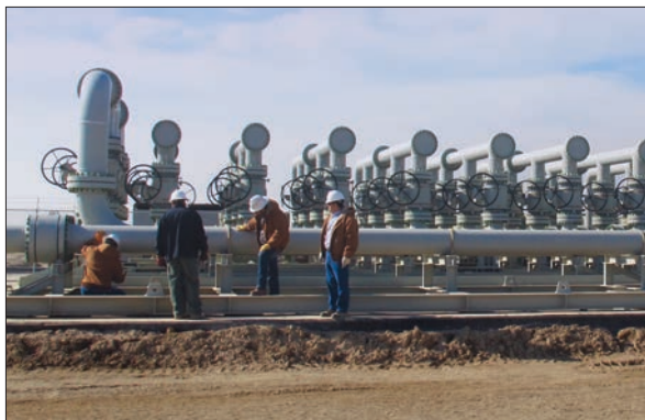
A new gathering system at West Qurna 1 provides additional manifolds and allows optimization of capacity utilization across three different degassing stations.
