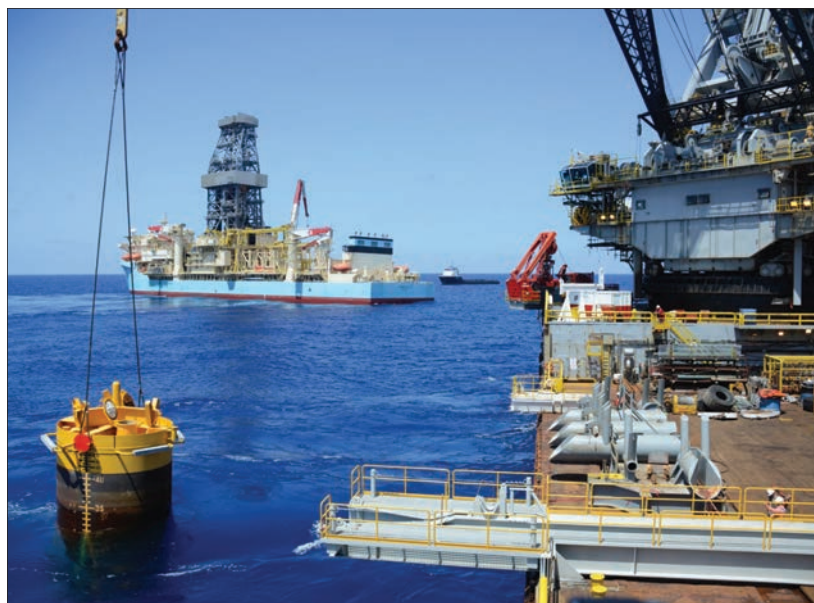
Subsea pile installation at the Julia Phase I project in the Gulf of Mexico.
