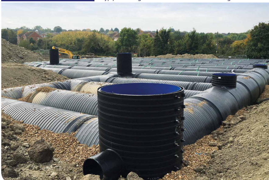
Polypipe's surface water attenuation solution for the Houghton Regis residential development scheme
