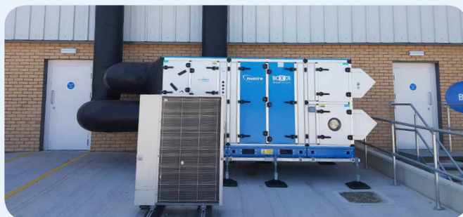
Nuaire Boxer Packaged Solutions (BPS) air handling unit
