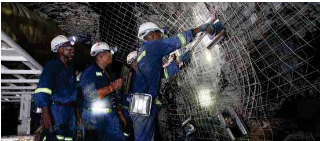
Lining the kimberlite tunnels with safety meshing.
